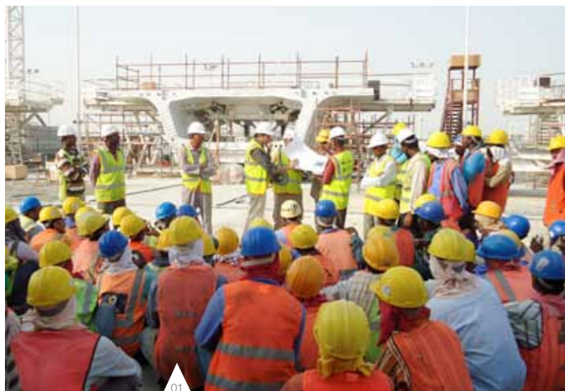
01 'Safety Time Out' meeting on the North Manama Causeway bridge site, Bahrain
